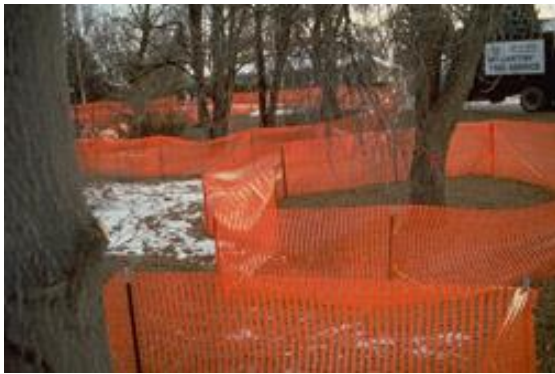
Figure 2. Example project Tree Protection Zone plastic barrier mesh fence
